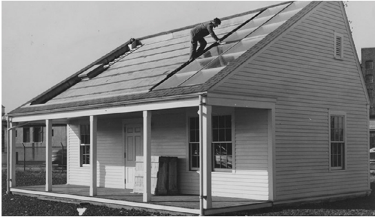
(clockwise from top left) Cars queuing for petrol in London during the 1979 oil crisis; the Saskatchewan Conservation House in Canada, one of the pioneering low energy houses of the 20th century, was built in 1977; constructed even earlier was the Solar 1 house at MIT, which was built in 1939, and featured 33 sqm of solar thermal panels and a huge storage tank to meet its heating demand.
