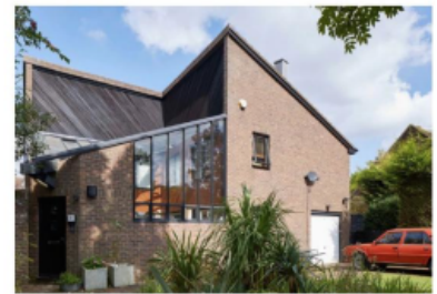
(above) Showcased in HomeWorld '81 , Future Home 2000 included a number of experimental approaches including an adapted car engine to run an electric generator with heat recovery.
