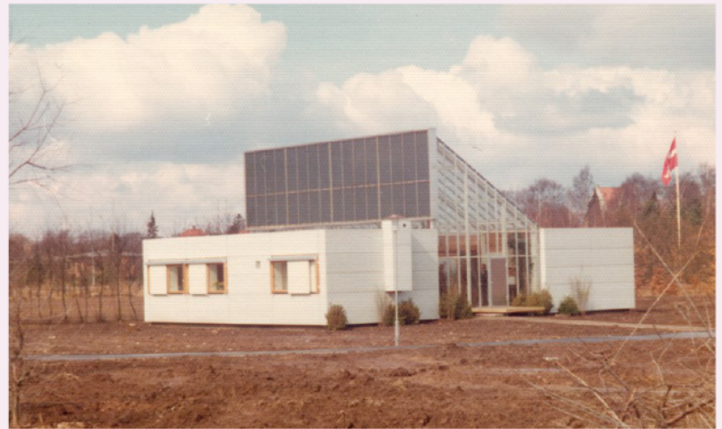
The Danish 'zero energy house', built in the aftermath of 1973-74 oil crisis.
